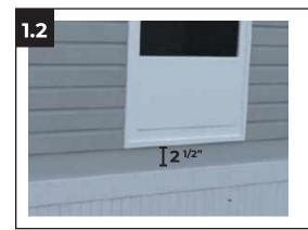
Once the area has been outlined, measure down from the top of the door threshold 2 1/2". This point will be a reference for the surface of the deck.
