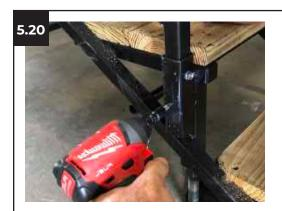
Once the **Step Handrail (O)** is seated firmly in position, secure with 14 x 14 x 3/4 Tek screws through the pre-drilled holes on both sides of each sleeve.
