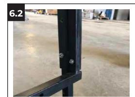
Secure each **H-Brace (C)** to the **Adjustable Legs (A)** with a second 14 x 14 x 3/4 Tek screw in the remaining pre-drilled pilot holes.
