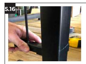
While holding the second **End Post (G-H)** in position, slide the other end of the **4 1/2" Deck Rail (N)** section into place. Repeat steps **5.4-5.5** to secure the post to the top of the deck.
