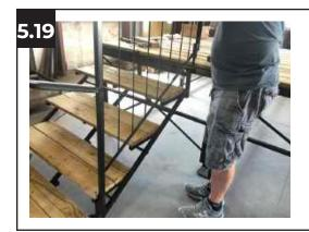
To attach the **Step Handrail (O)**, position it above the outside of the Step Assembly and slide the male connectors down into the sleeves (located on the back of the top step tread and the front of the second step tread).
