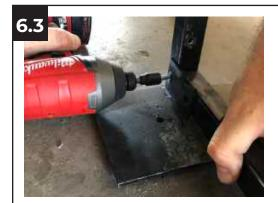
Finally, use 14 x 14 x 3/4 Tek screws to attach each **H Brace Support (Q)** on the interior of the 48" side of the deck frame.
