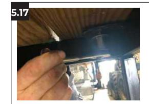
After ensuring all posts and deck rails are plumb and mounted correctly, tighten down all Carriage Bolts installed in this section.
