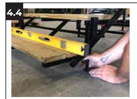
Place a carpenters level across the bottom step tread and turn the **Adjustable Step Legs (F)** until level. Verify the top step is level in both directions.
