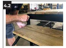
Move the top of the **Step Assembly (E)** against the deck frame so the pre-drilled holes on the attachment plate (located on the back of the top step tread) line up with the pre-drilled holes in the **Platform Module (D)** frame.
