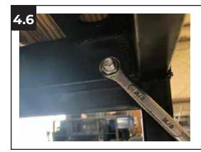
After confirming the **Step Assembly (E)** is level and step height is verified, tighten down the nuts from step **4.3**.
