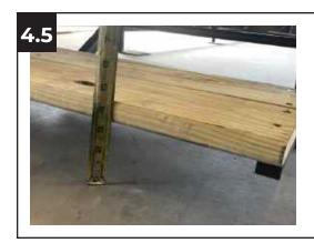
Verify the height from the ground to the top of the first step tread does not exceed 7 3/4"(the maximum height adjustment allowed).
