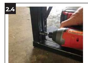
Secure both Connector Braces (B) to each H Brace (C) with a  $14 \times 14 \times 3/4$  Tek screw.
