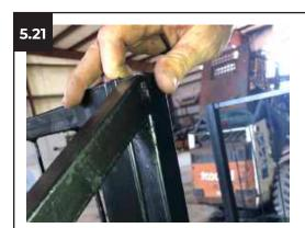
Hold the **Step Handrail (O)** in place so it is flush with the front of the **End Post (G-H)** mounted in step **5.16**. Secure the **Step Handrail (O)** to the **End Post (G-H)** with a #10-16 x 3/4" Phillips head screw through the pre-drilled pilot hole located in the top of the post.
