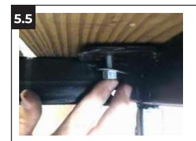
On the underside of the deck, slide a washer onto the carriage bolt and secure with a nut. Hand tighten, leaving allowance for adjustments.
