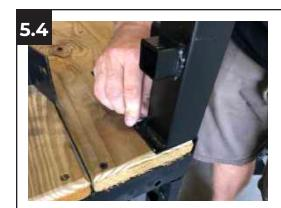
Insert a 2" x 3/8" Carriage Bolt through the hole in the top of the post bracket and the newly drilled pilot hole.
