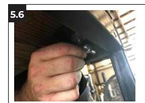
Repeat this process using a 1 3/4" x 3/8" Carriage Bolt through the hole in the front of the post bracket.
