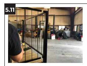
Insert the 44" Deck Rail (L) section into the sleeves located on the side of the second Corner Post (J).
