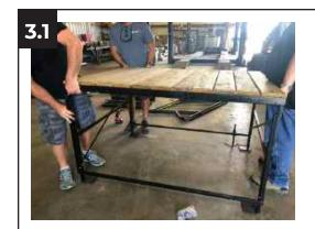
Move the **Platform Module (D)** into position above the frame of the deck and slide the male connectors down into the top of the **H Braces (C)** until it is seated securely on the frame.
