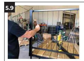
While holding the second Corner Post (J) in position, slide the other end of the 58 3/4" Deck Rail (K) section into place. Repeat steps 5.4-5.6 to secure the post to the top of the deck.
