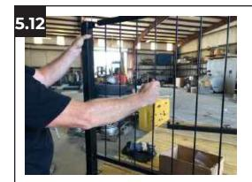
While holding the first **End Post (G-H)** in position, slide the other end of the **44" Deck Rail (L)** section into place. Repeat steps **5.4-5.6** to secure the post to the top of the deck.
