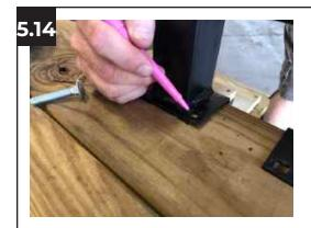
Once positioned correctly, mark the location of the hole on the top of the post bracket. Use the mark as a guide to drill a pilot hole through the **Platform Module (D)**. Once drilled, reposition the post in place.
