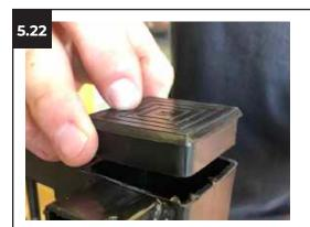
After all deck rails and step rails have been properly secured, install the 2" x 2" post caps in the top of each post.
