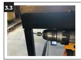
After leveling, secure the **Platform Module (D)** to the **H Braces (C)** with one 14 x 14 x 3/4 Tek screw in the pre-drilled holes located on the top of the **H Brace (C)**.
