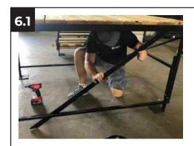
Using  $14 \times 14 \times 3/4$  Tek screws, attach each **Cross Brace (P)** on the interior of the 60" side of the deck frame.
