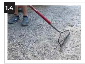
After verifying all measurements are correct, smooth out the area as much as possible before beginning installation, allowing for 1/2" slope of ground elevation for every 12" of distance from your home.
