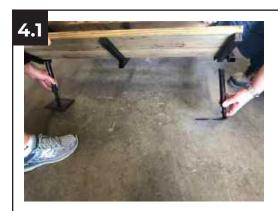
Move the **Step Assembly (E)** to your desired location (left or right side of the deck). Raise the top of the **Step Assembly (E)** vertically and slide the **Adjustable Step Legs (F)** inside the sleeves located on the bottom step tread.
