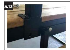
Position the second **End Post (G-H)** so it is seated next to the **Step Assembly (E)** (on the side furthest away from the home) ensuring the front of post bracket is flush with the attachment plate on the **Step Assembly (E)**.
